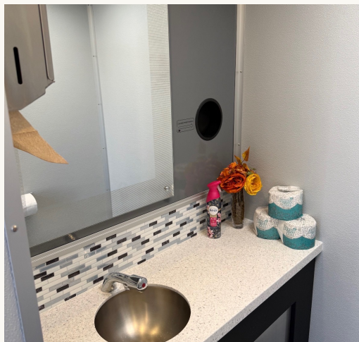
Vanity & interior finishes
